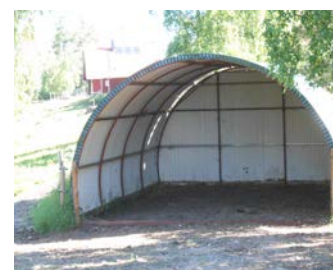
Pic 43. A wind shelter made from metal sheets on a steel frame can be moved shorter distances by lifting it with a tractor inside.
