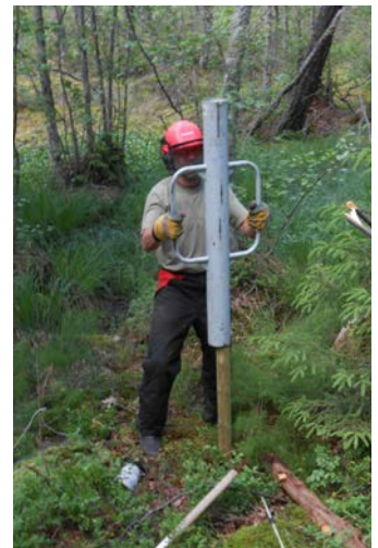
Pic 36 A man killer is used to bang down fencing posts.
